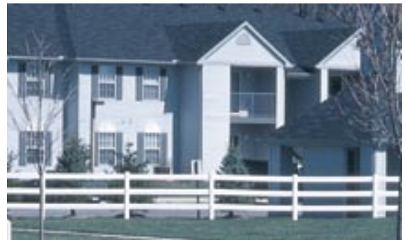
Three rail around an apartment complex
